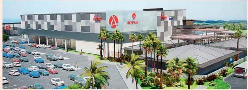
Gateway Palmerston's 37,000m<sup>2</sup> of roof area will contain 1.5 megawatts of solar panels.
